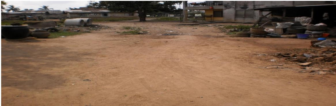
Plate 7: Access road to each dwelling without drainage system cause havoc during the raining season
