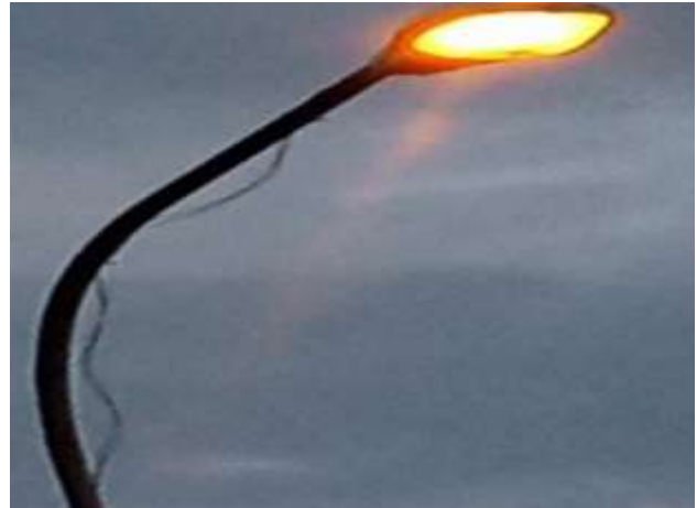
(b) High Pressure sodium light as street light
