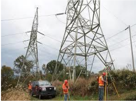
Figure 10: Surveyors mapping power transmission lines
