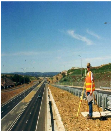
Figure 3: Surveyor on a road project:
