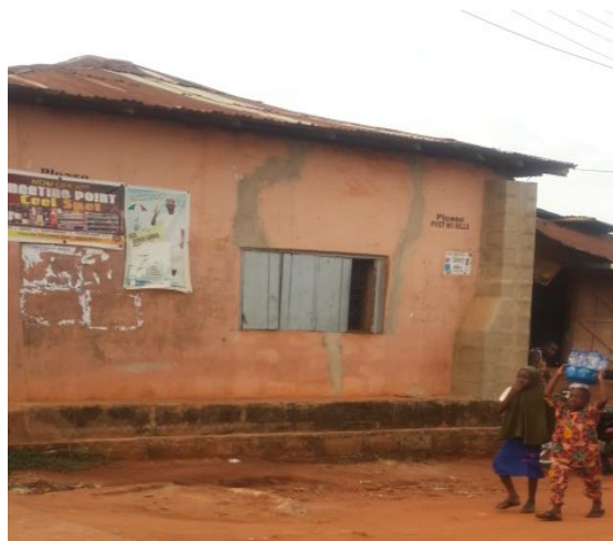
Plate 14, Classroom building at Library area completed Completed in less than 10 years. Badly affected by weather Source: Authors field photograph 2017.
