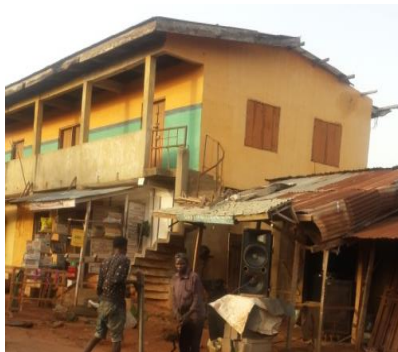
Plate 2 Commercial building at Orita Oja Odan road Completed for over 20 years fairly affected by weather Source: Authors field photograph 2017.
