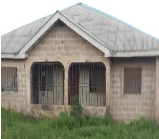
Plate 11 Residential building with Unplastered block wall in use for less than 10 years at Express road.
