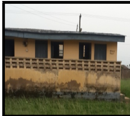
Figure 12: Public Toilet at Federal Polytechnic Ilaro Completed in Less Than 10 Years, Badly Affected by Weather Source: Authors Field Photograph 2017
