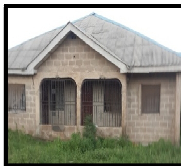
Figure 10: Residential Building with Unplastered Block Wall in Use for Less Than 10 Years at Express Road
