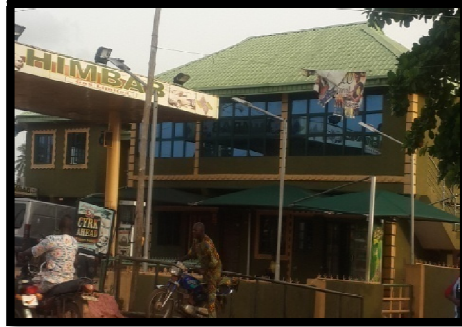
Figure 8: Commercial Building with Glass/Painted/Wall Finish along Library Area Rehabilitated within The Last 10 Years
