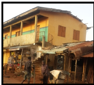
Figure 3: Commercial Building at Orita Oja Odan Road Completed for Over 20 Years fairly affected by Weather Source: Authors Field Photograph 2017
