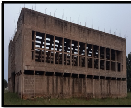
Figure 11: Sport Centre Unplastered Block Wall Abandoned For Over 40 Years at Federal Polytechnic Ilaro. Badly Affected by Weather Source: Authors Field Photograph 2017
