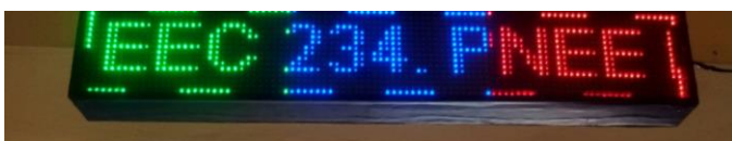
Figure 8c. Installed Laboratory digital timetable display
