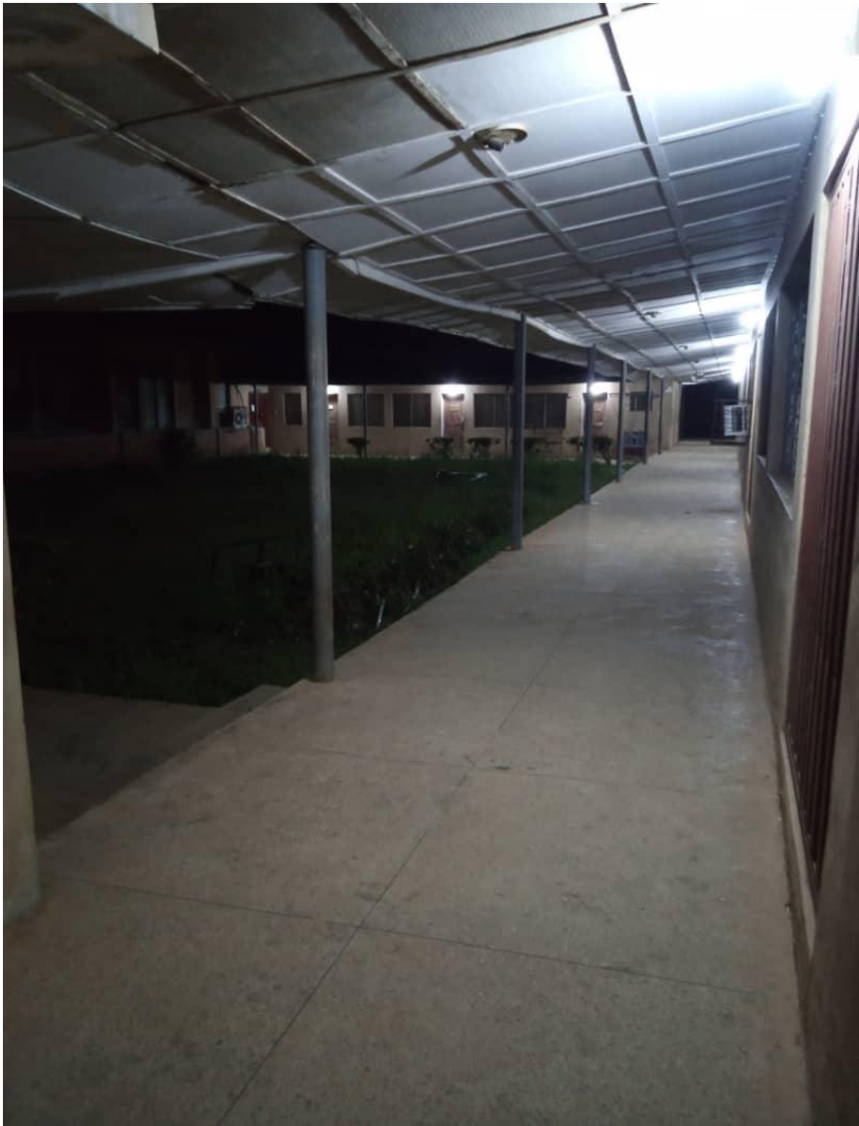
Figure 12: Lighting condition of the walkway at 06:50 PM
