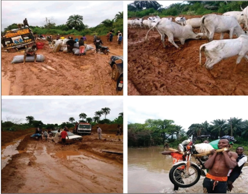
Figure 1. Pictures Depicting the Deplorable Condition of the Road Leading to Kurmi Local Government Area of Taraba State, North Eastern Nigeria
