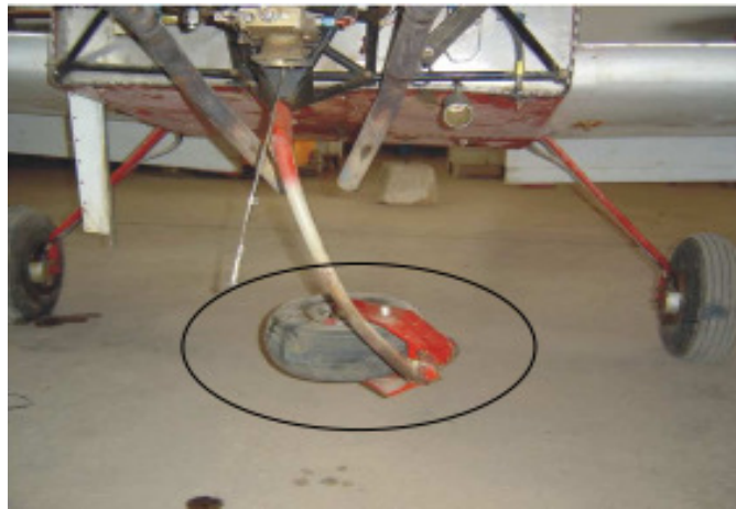
Plate 1: The Failed Strut
