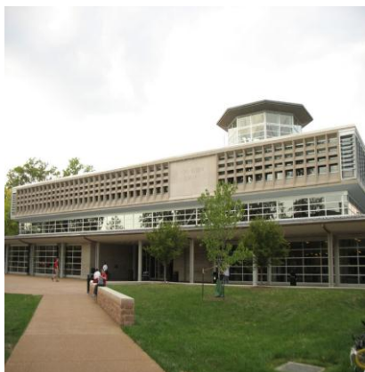
Fig. 5 Washington University Library as examined by Wilson (2012) before rehabilitation for sustainability Source: Internet Google Search
