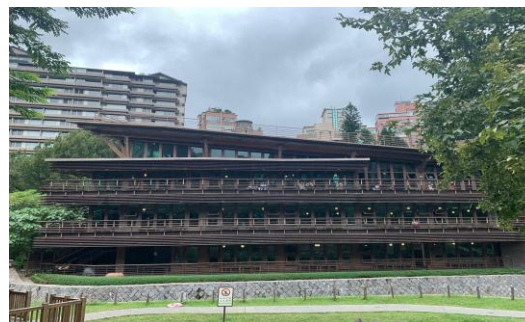
Fig. 4 Side view of Beitou Public Library in Taipei as evaluated by Tseng (2007) for sustainability
