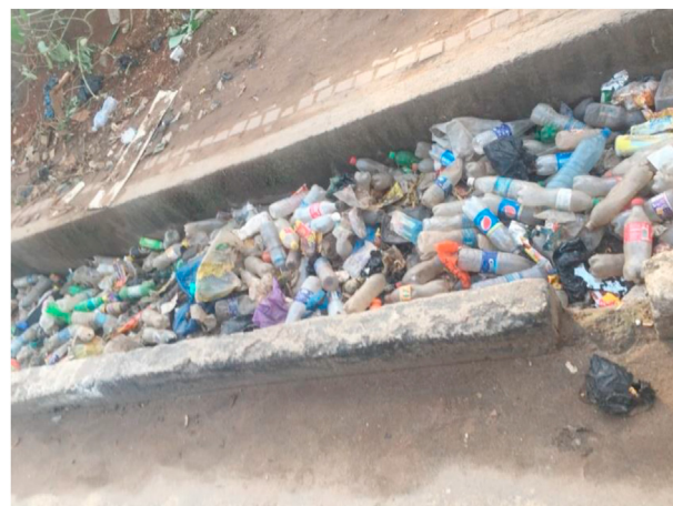
Figure 1. Plastic waste blocking drains.
