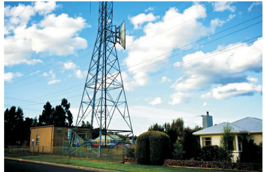
Plate 2.1: A tower located too closely to a high tension power line and a residential building
